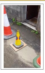
Repairs to our water supply in winter meant the path to the north door was dug up. Everything was fixed and refilled but then the very dry weather meant one of the repairs collapsed creating a small sink hole with some very bendy tarmac.
